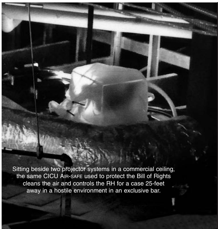
Sitting beside two projector systems in a commercial ceiling, the same CICU AIR-SAFE used to protect the Bill of Rights cleans the air and controls the RH for a case 25-feet away in a hostile environment in an exclusive bar.
