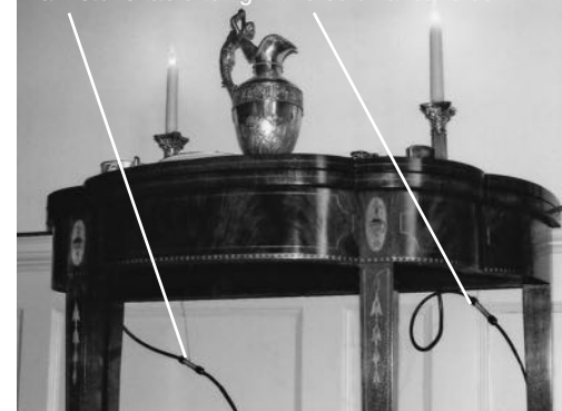
DMSPs connect 3 mm fiber to 1 mm fiber under a historic table to light two colonial candles.
