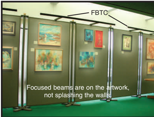
Temporary walls cover windows with FBTC tracks mounted on top.
